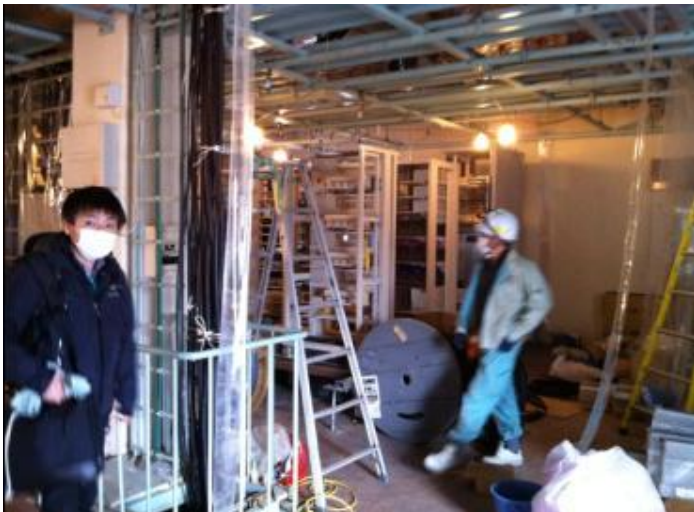
Construct rack facilities
